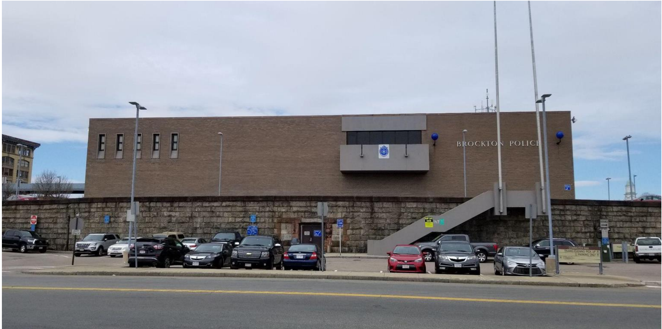
Brockton Commuter Rail Station and Police Station
