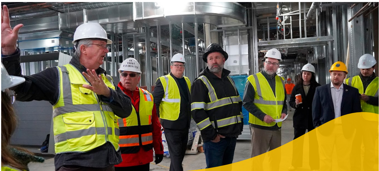
Leaders tour the new Congdon-DeValles school under construction in New Bedford’s Goulart Square neighborhood.
